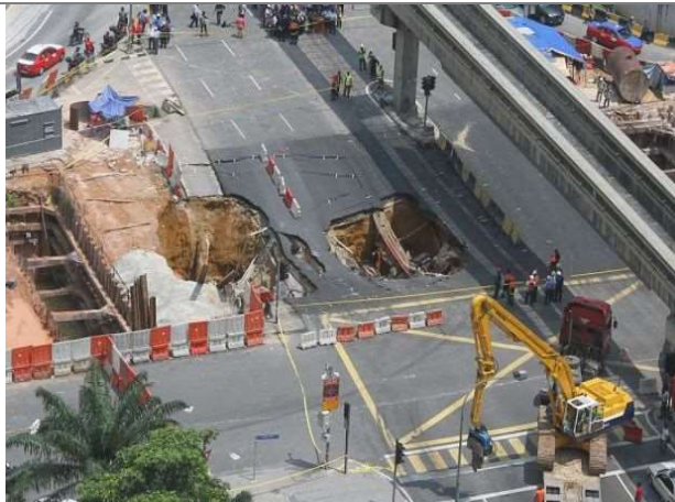
Sinkhole on existing road due to excavation works
