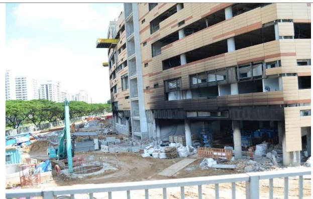
Fire damage to building under construction
