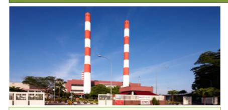
Incineration plants are also known as waste-to-energy (WTE) plants. The heat from the combustion process is used to generate superheated steam in boilers. The steam is in turn used to drive turbogenerators to produce electricity.
