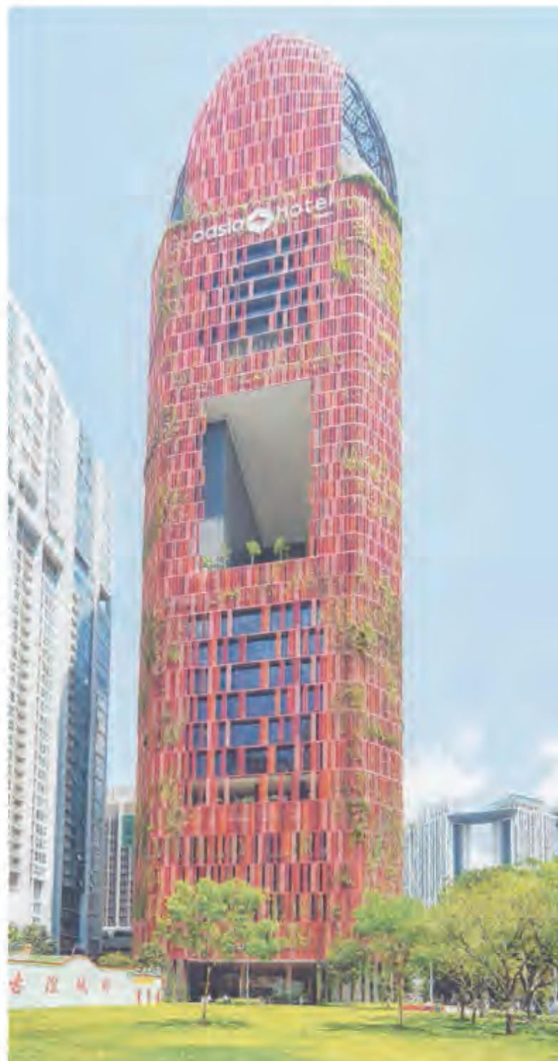
Dasia Hotel Downtown was designed by Spanish designer Patricia Urquiola with local firm WOHA. The new law will allow foreign architects from participating jurisdictions to practise here. ST FILE PHOTO
